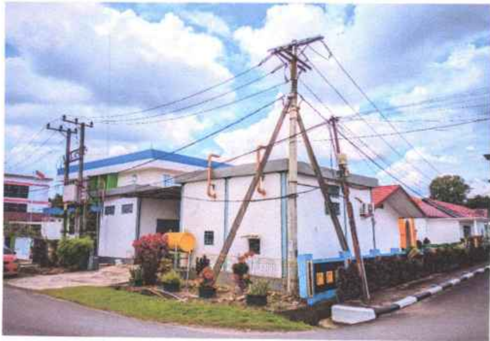
Gambar 2.9 Gedung Power House
