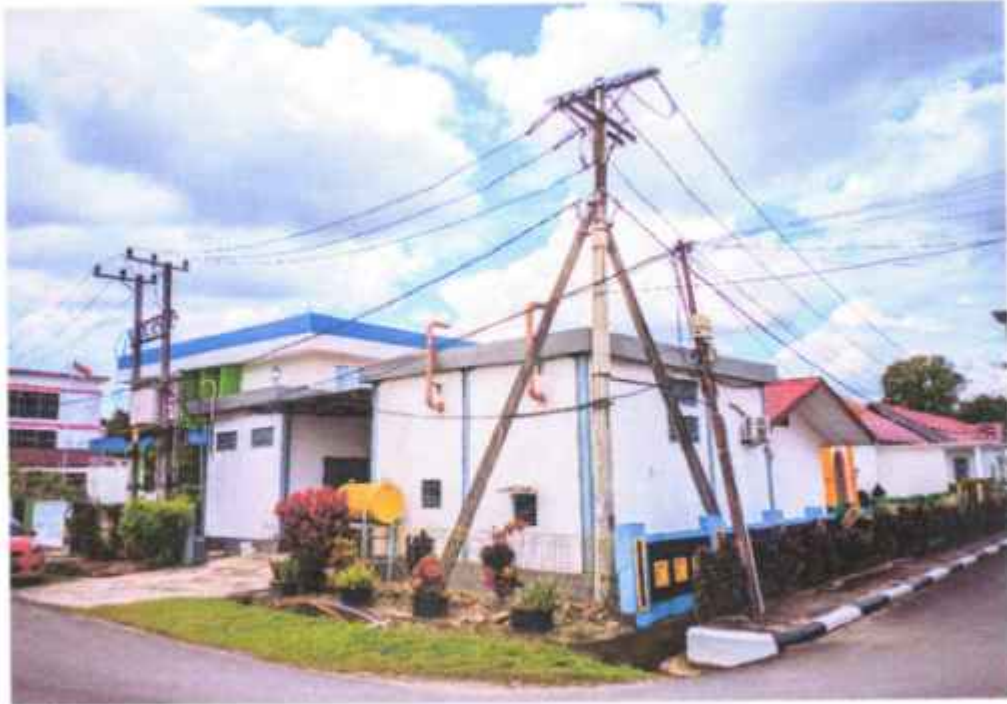
Gambar 2.9 Gedung Power House
