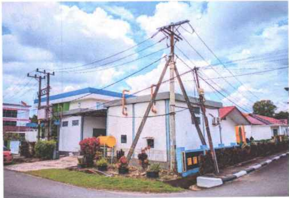
Gambar 2.9 Gedung Power House
