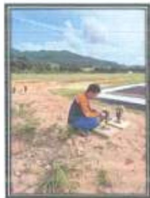
Ganti Lampu Bohlam Threshold
