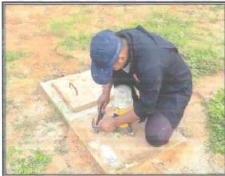
Pemasangan skin Grounding Runway
